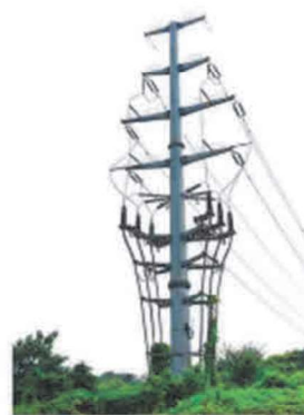
终端电力杆 Terminal power pole
